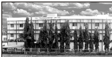
Corporate Office & Works (J-7, Hingna, MIDC)
